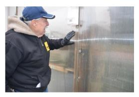
an end wall panel that had blown off the shelter due to high winds. Perry Straw, Dave Barrows and Bruce Andresen were able to re-secure the same panel to the shelter, as most of the fasteners in the wood pulled out due to rusting of the threads or decayed wood. The fasteners in the pipes have very small washers, and the panel pulled itself thru the fastener hole. By placing a much bigger washer on the latter fastener, those
